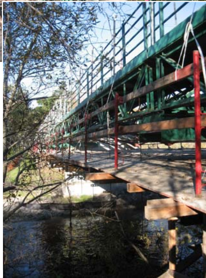
Above: Rancho San Carlos bridge getting its roadbed replaced, and repainted, by end of May, 2011
